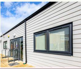
The finished building offers modern and high-spec teaching and SEND facilities plus a host of future-proofing sustainable features. Aesthetically, attractive light grey Cedral cladding finishes the external façades of the modular classroom unit and ensures the new building complements the existing school blocks.
